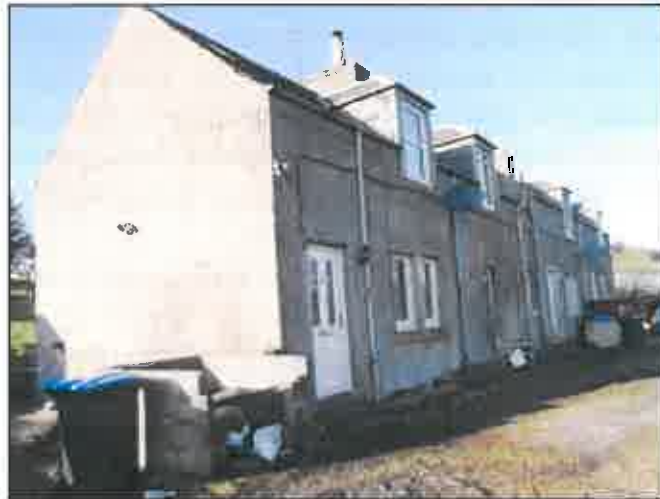
Fig 1: Front elevation of 3 Wormiston Cottages with bedroom upstairs:
