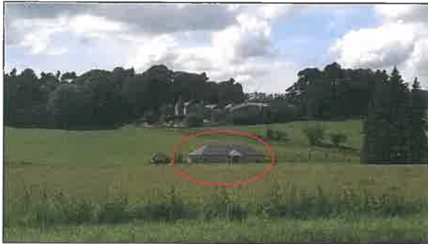
Fig 20: Bungalow at Darnhall Farm, Eddleston
