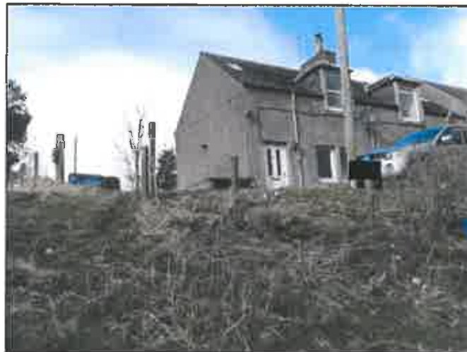
Fig 7: View of southern elevation
